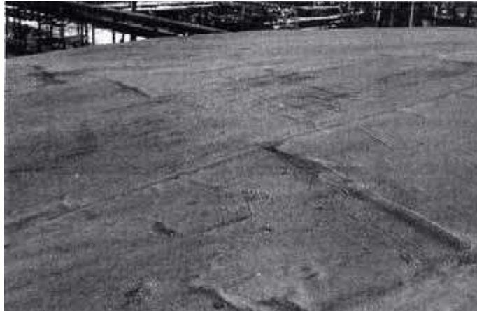
Figure 6-28 bitumen roof coverage
