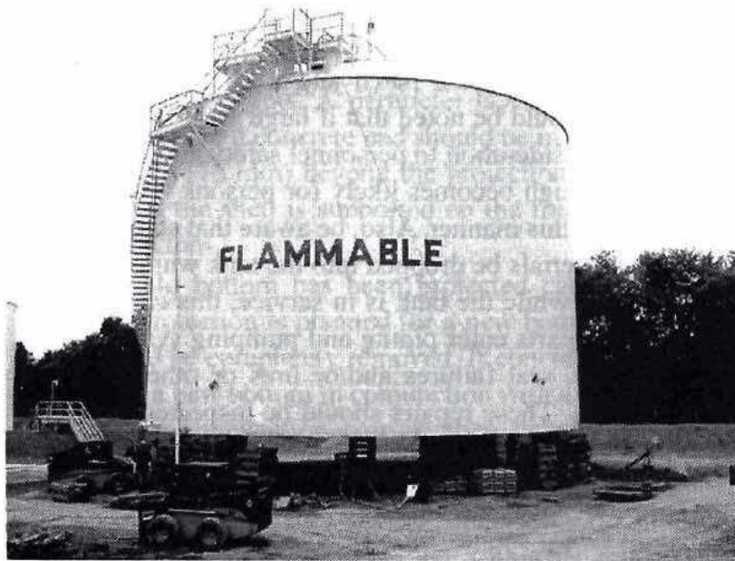
Figure 6-19 Lifted tank to repair below layer
